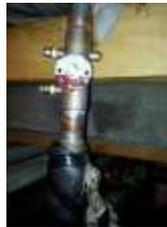
PH traps are serviced annually to help neutralize acidic discharge from the high efficiency boilers. The systems have simple traps that are basically 2" pvc pipes filled with marble chips. There is room for improvement and we should consider adding larger traps that contain more marble and would better neutralize the discharge, which eats away at cast iron sewer lines.
